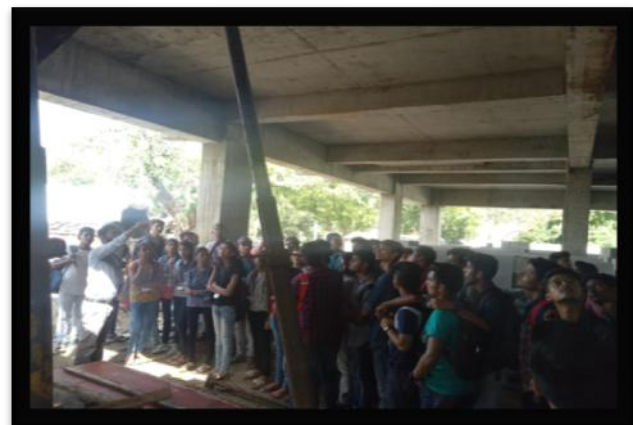
Post Tension Slab Casting, St. John college of Humanities and science, palghar, B.E CIVIL 23 rd March 2019
