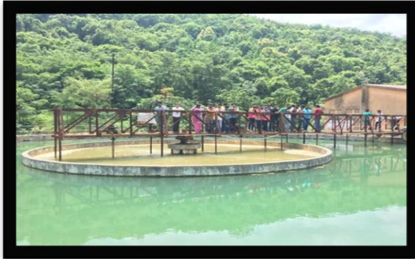
Water Treatment Plant, Shelwali Dist. Palghar, B.E CIVIL on 21th September 2019
